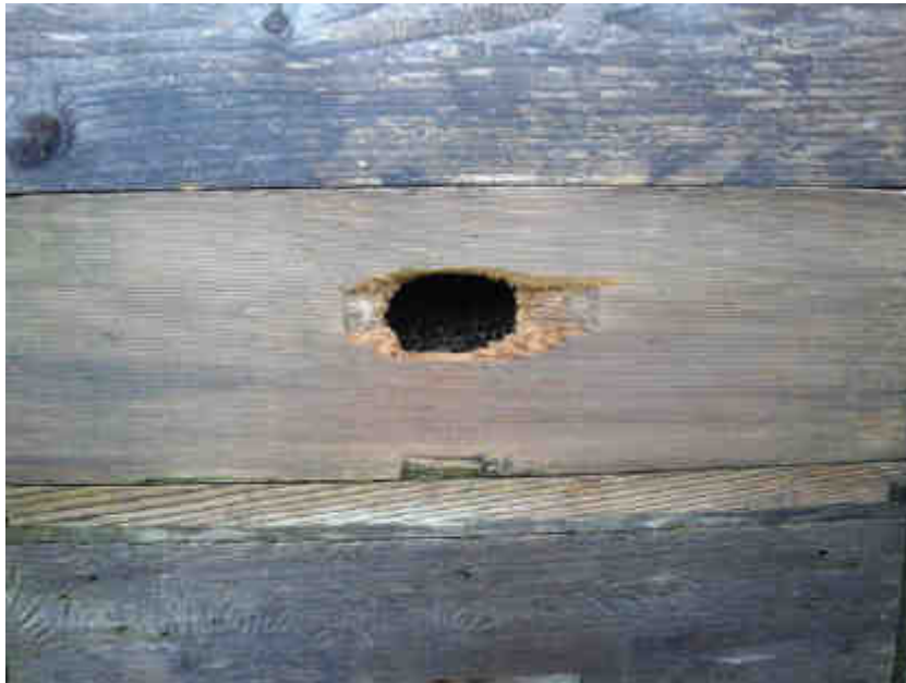
Woodpecker damage at the Water Mill Apiary Photo courtesy of Tony Mabey
